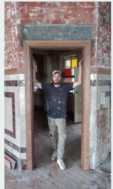
one of our amazing team with the freshly renewed door frame - post flood repairs
