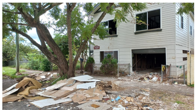
“Mazzer House” in Casino Street, during the first cleanup
