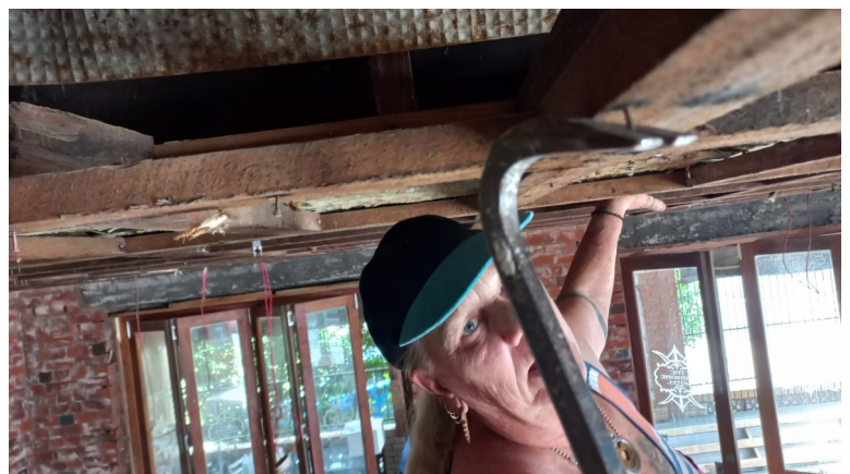
"Leanne, doing her nails" The ceiling in the bar had to be removed, and every nail in the existing frame, removed
